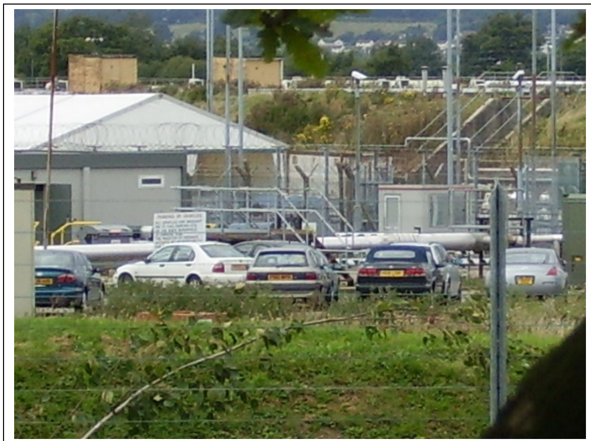
Figure 3. Tents and temporary portacabin accommodation in the car park adjacent to the nuclear licensed site area at AWE Burghfield, August 2007. The tents were used to process, inspect, and clean items from flooded buildings, using radiological protection contamination control principles to segregate ‘clean’ and ‘dirty’ items.
