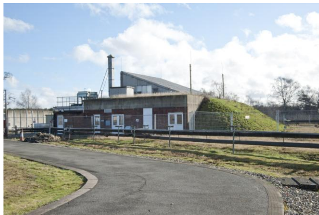
External view of the building after the fire
