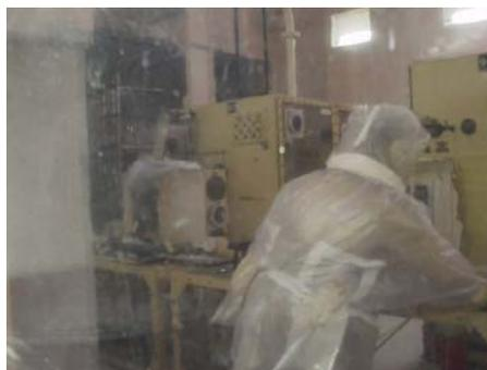
**PBAS size reduction of glovebox and transfer tunnel**
