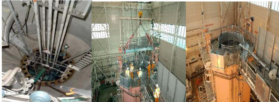
**1 Reactor with water level lowered and lattice plate visible**
