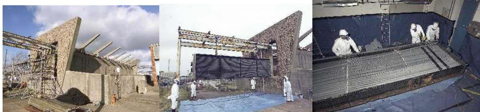
**1.ABR structure prior to decommissioning work    2. Removal of radiators    3. Cutting radiator pipes into small lengths**
