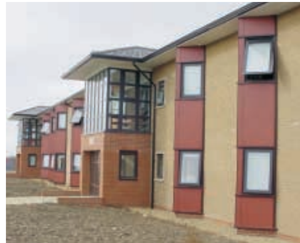
MOD is undertaking the largest ever programme of work to upgrade Service accommodation.
