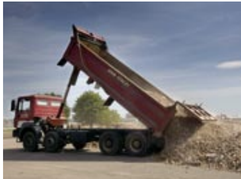
Graded material from demolition is stored on site for re-use
