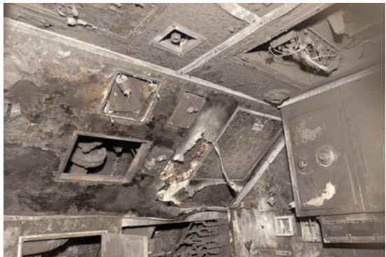
Fire damage to HMCS Chicoutimi (formerly HMS Upholder)
