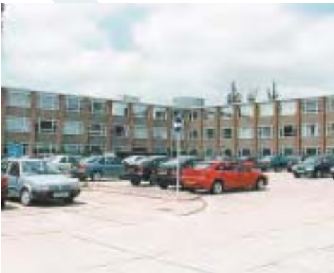
Internal Courtyard Space.
