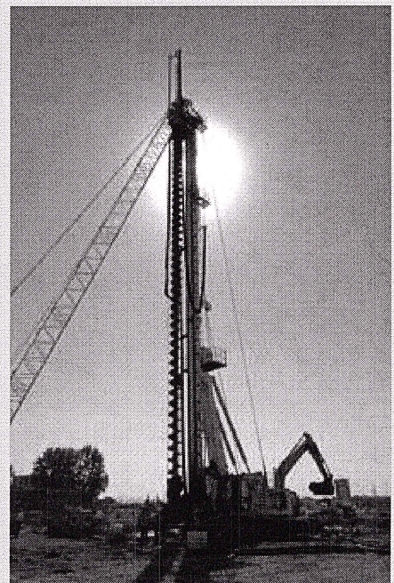
Sinking of over 300 piles, up to 30 metres deep, commenced in August 2006
