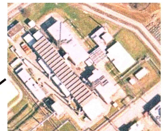
A45 Manufactures HEU components. Area to be refurbished.
