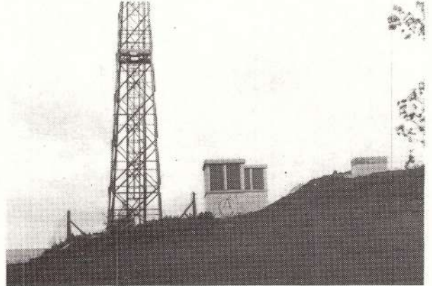
Ventilators at Skipton, Yorks. 'T' shaped bungalow is nearby.
