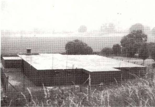
Surrey Police control centre. A X headed bunker — unique as cross-headed aerials are located elsewhere (nearby)
