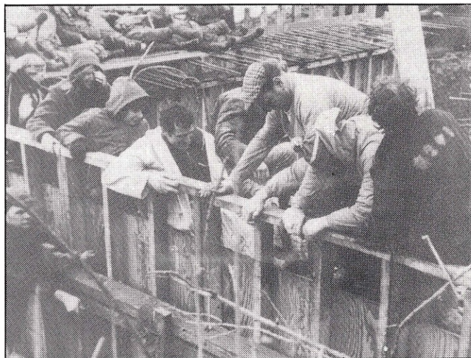
Peace campaigners obstruct contractors pouring concrete during the building of Mid-Glamorgan County Wartime HQ.
